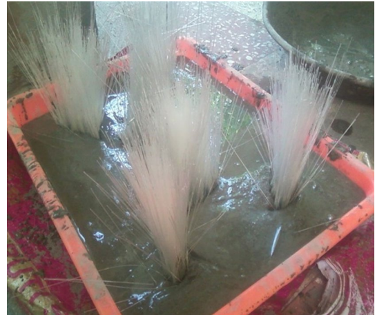
Fig. 5. Placement of optical fibers
